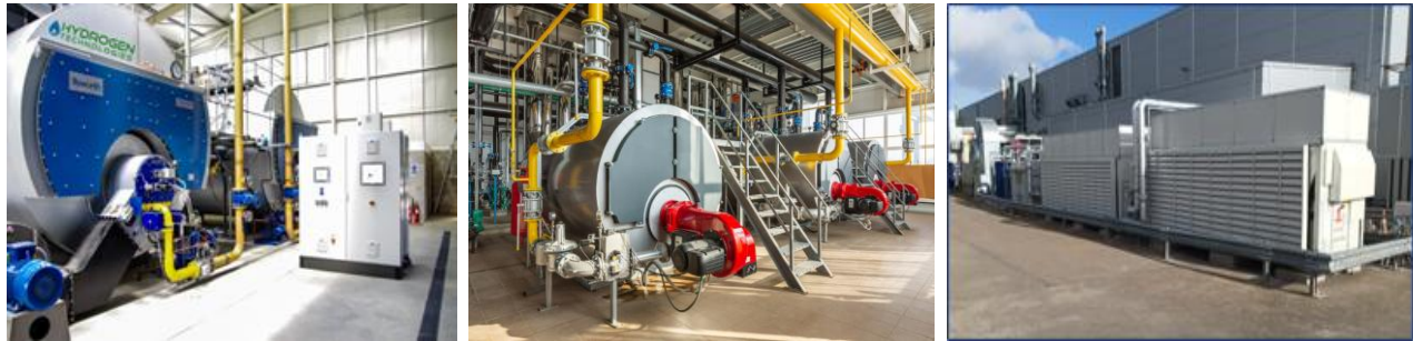
ITP Aero air source heat pump powered AHUs at the Hucknall site.
